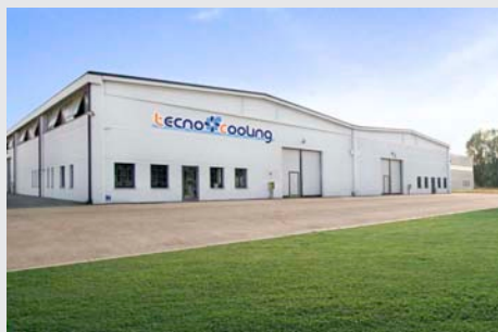
Stabilimento 2 - Castelnovo factory
